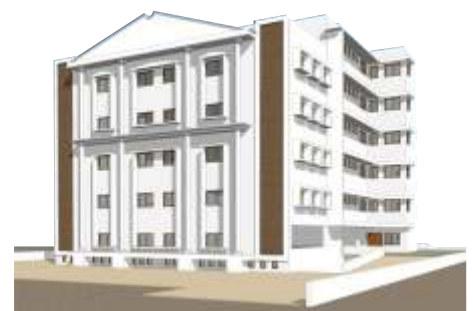
Mihan SEZ, Nagpur (under construction)
